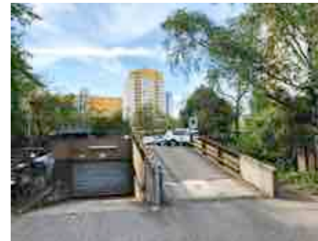
Parkdeck in der Obstallee
